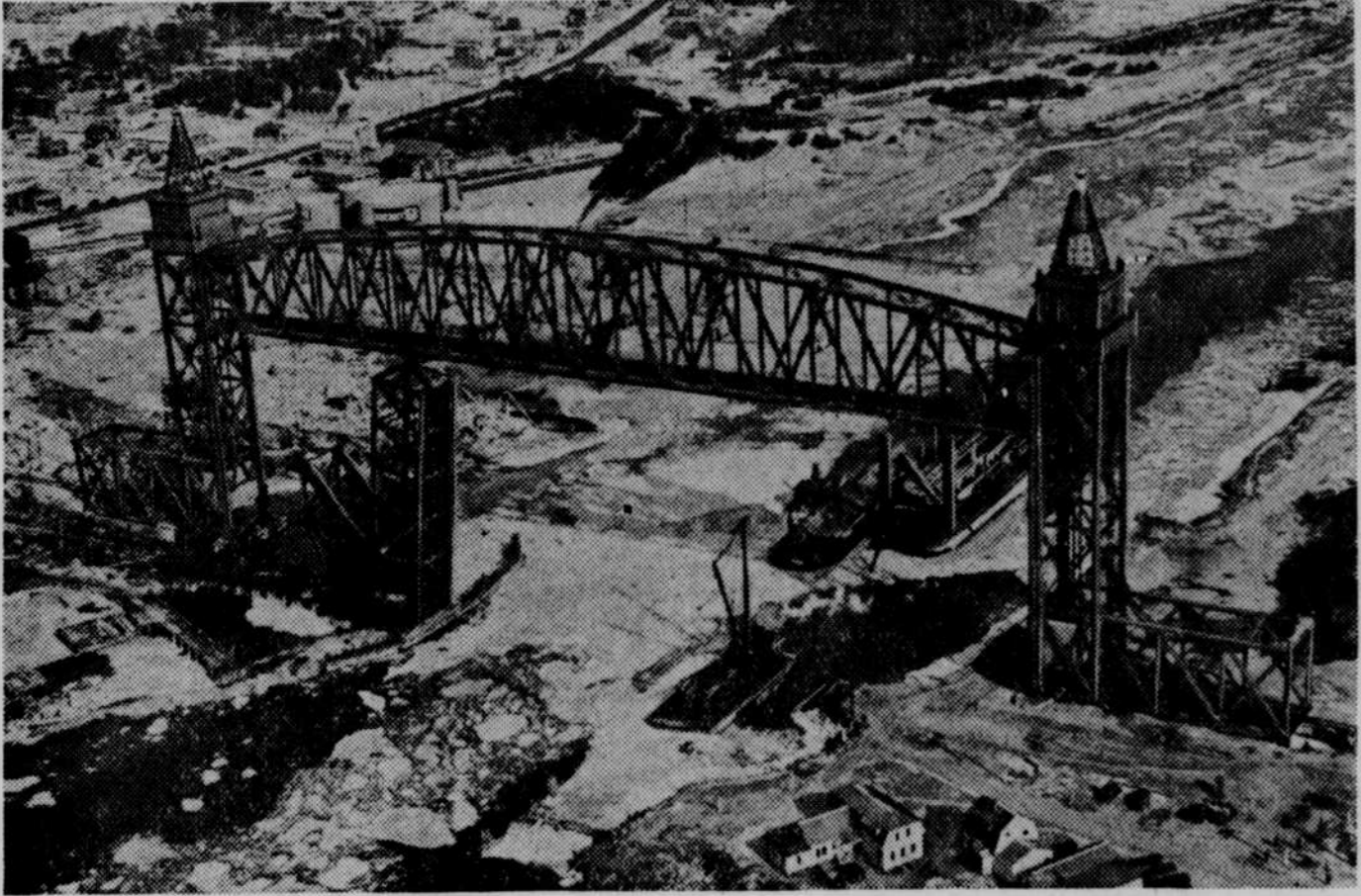
This photograph, made from a plane over the new vertical type lift railroad bridge spanning the Cape Cod canal, shows just how greatly hampered shipping was in the canal due to huge cakes of ice. Only the largest vessels could pass through.
