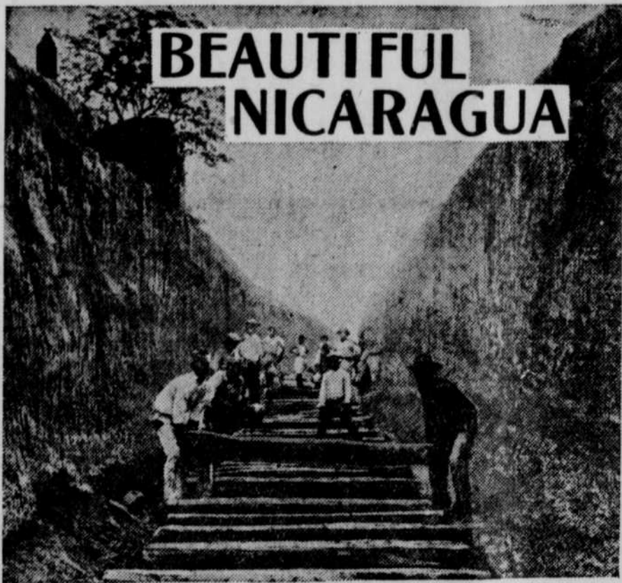
Railroad Building in Nicaragua.
