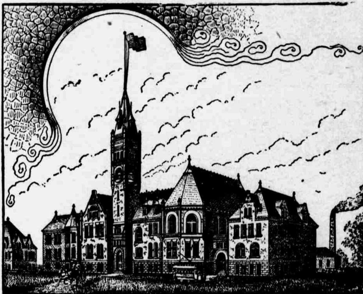
Main Building. 265 Feet Front.
