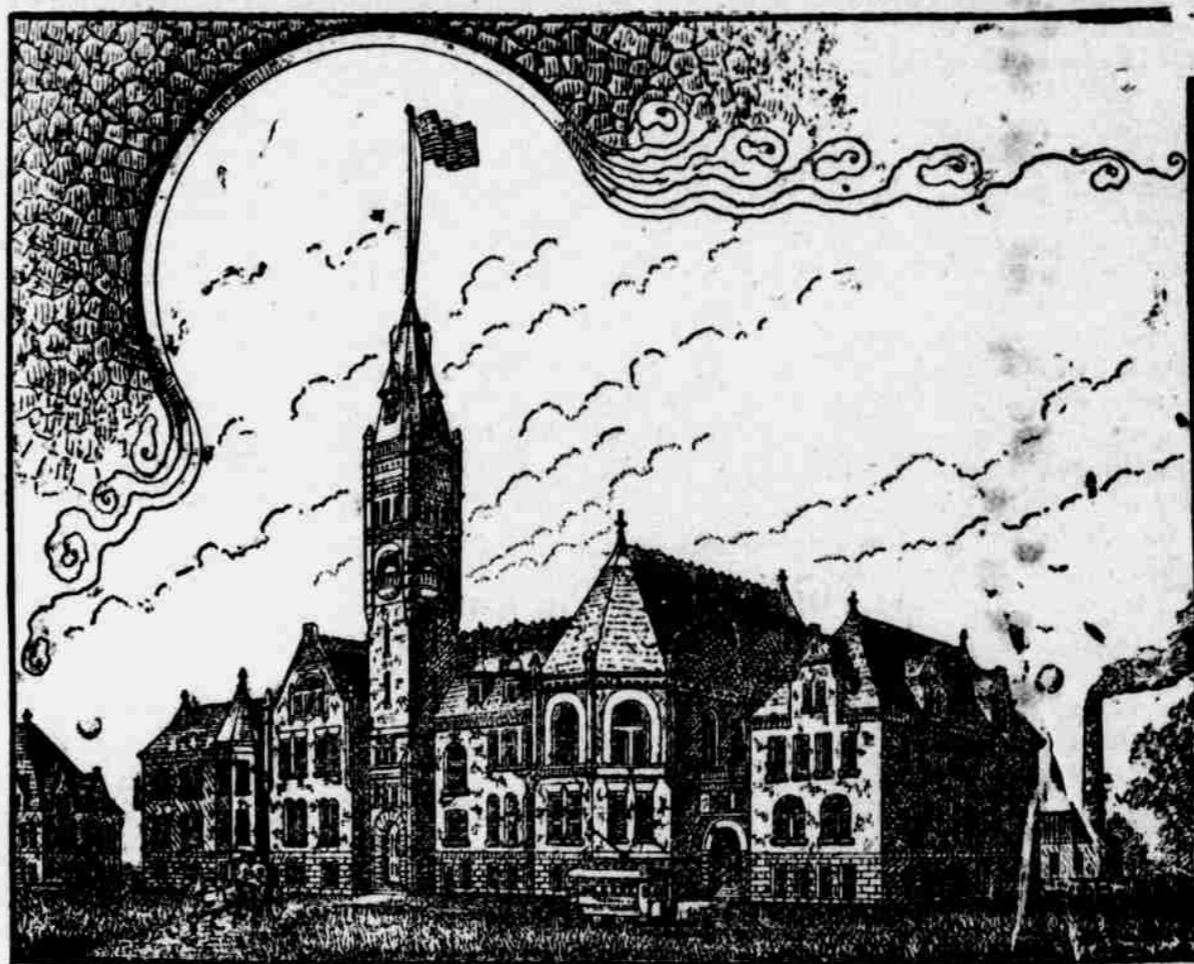
Main Building, 265 Feet Front.
