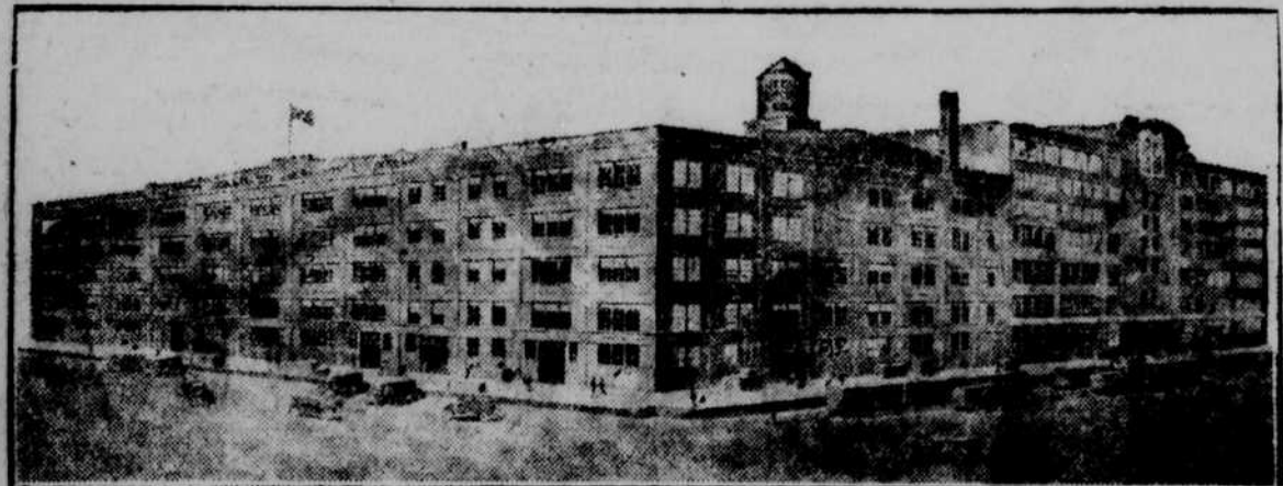
CAPITOL AVENUE, TWELFTH TO THIRTEENTH STREETS
