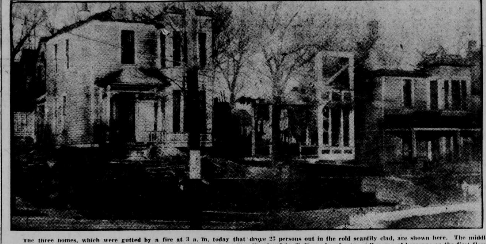
The three homes, which were gutted by a fire at 3 a. m. today that droye 23 persons out in the cold scantily clad, are shown here. The middle house, which is totally destroyed, was where the fire started and where Fire Warden John T. Dunn found a two-gallon can of kerosene on the first floor.
