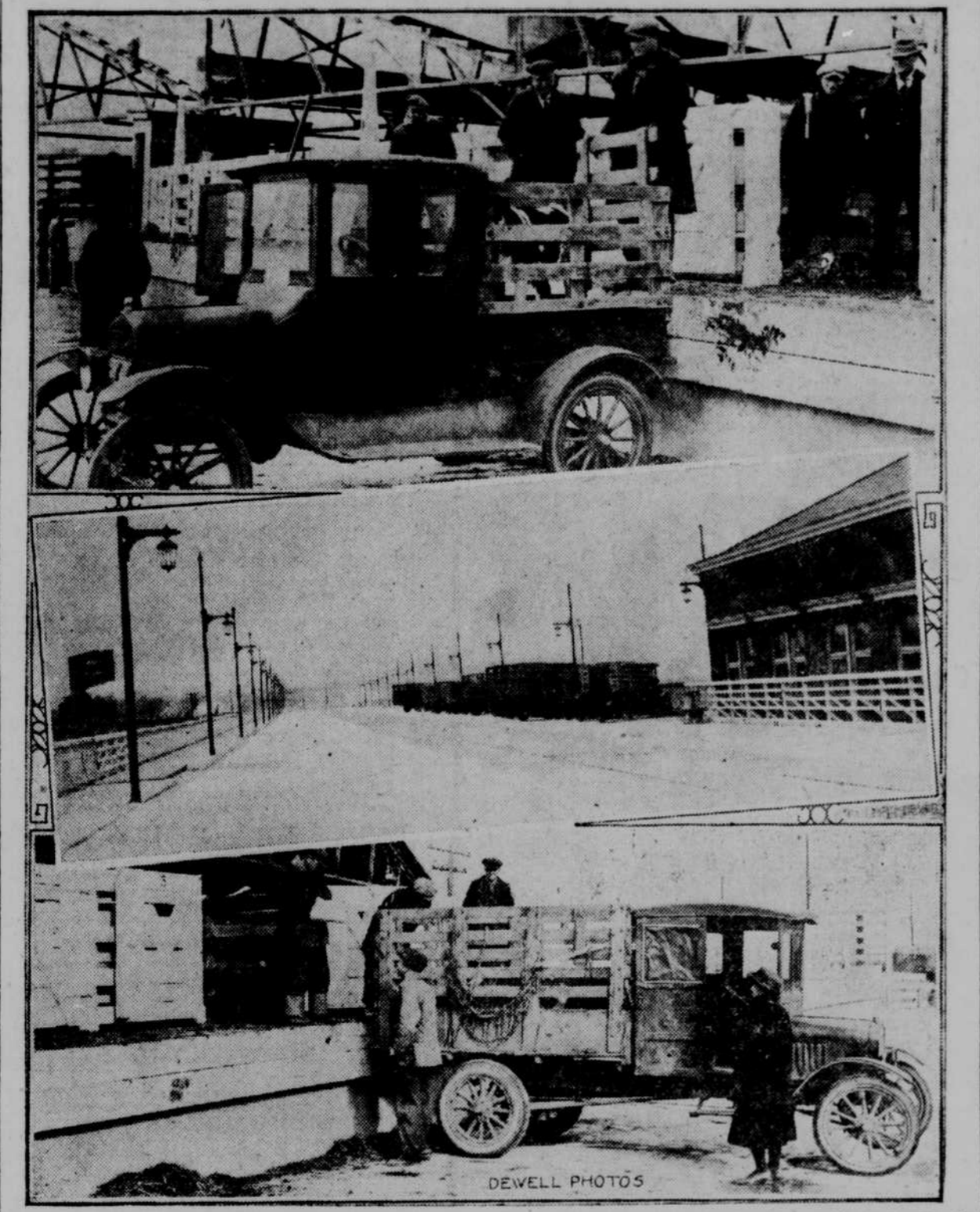
The Union Stockyards will today open its new unloading chutes for stock arriving by truck at the Omaha market and its newly completed viaduct, erected at a cost of more than $500,000. The above pictures show the new chutes and the north section of the viaduct. The top picture shows Albert Watumus of Chalco, Neb., ready to unload his stock into the trench pens, where truck stock is held preparatory to being weighed and consigned to a commission merchant. Lower picture gives a view of another section of the chutes, with L. E. Scholing of Springfield, Neb., having his stock checked before unloading. The two loads of stock were the first to be unloaded at the new chutes as well as the first trucks to cross the viaduct.
