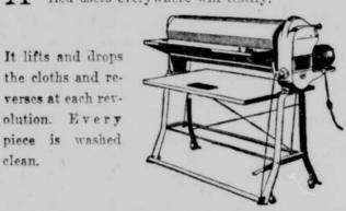
Constructed entirely of metal with an aluminum wringer and cylinder. 10 sheet ca-
