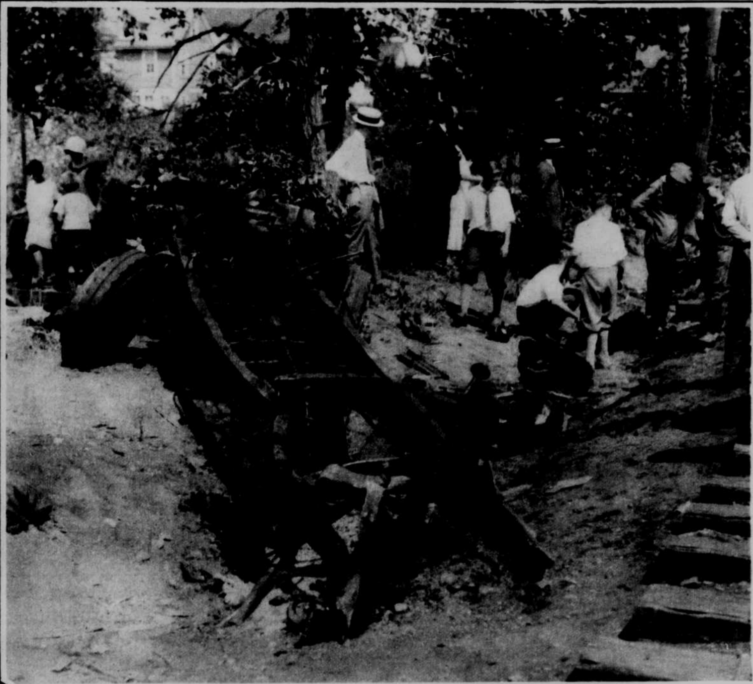
Crack Reading Express wrecked at Cranford, N. J. Traveling at sixty miles an hour, it struck a heavy truck, tore up the roadbed for 500 feet, and rolled down a small embankment. The engine and 3 of its four cars turned turtle. Four men were killed and twenty were hurt. —Wide World.
