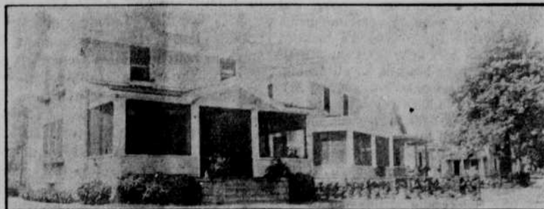
Glimpse of pretty block on Maple Street, west of Twenty-fourth, showing handsome residences of Joseph LaFour, Robert T. Walker, and Mrs. E. Howard.
