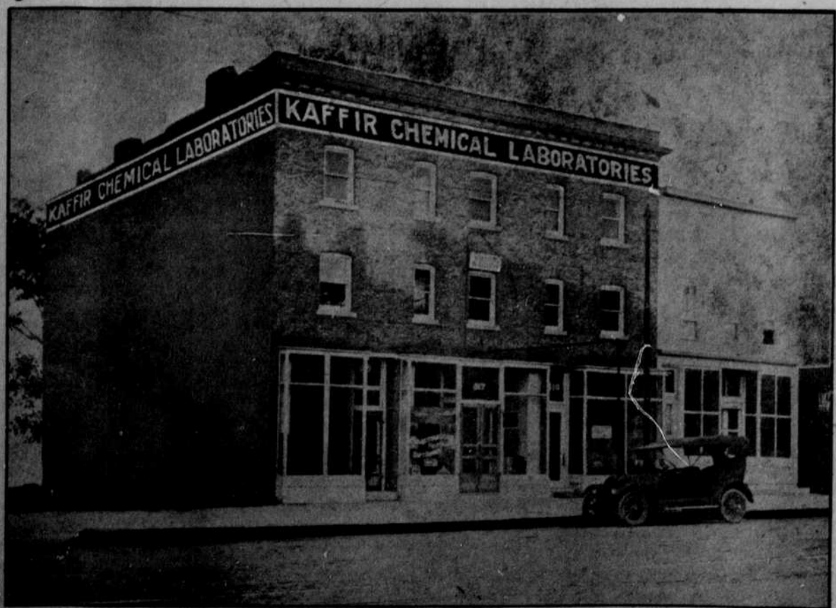
Home Building Kaffir Chemical Laboratories, Omaha, Nebraska
