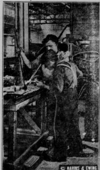
The highest grade of workmanship is required in the preparation of metal parts for airplanes. Every part must be finely tempered and accurately fitted to prevent collapse under hard strains. These men are welding parts of a navy hydroplane. The navy is guarding carefully publication of any parts or the whole of a finished plane.
