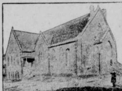
GROVE METHODIST CHURCH 22nd and Seward Sts., Omaha, Neb.
