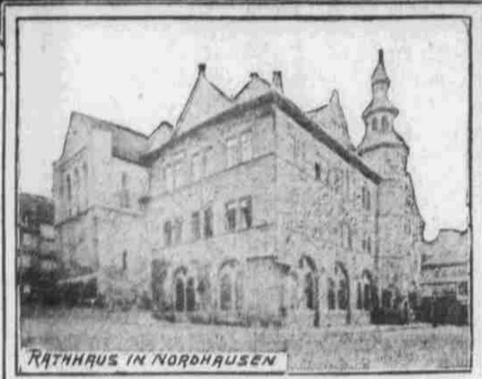
RATHHAUS IN NORDHAUSEN
