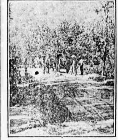
From Good Roads Magazine, New York. GRADING THE HIGHWAY
