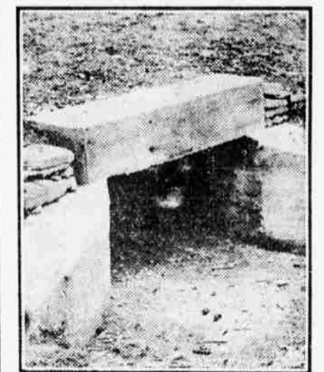
A CONCRETE CULVERT.
