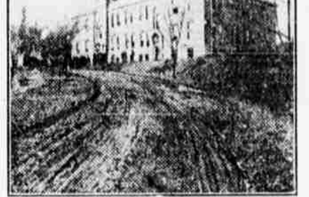
CONDITION OF A ROADWAY BEFORE USING DRAG.
