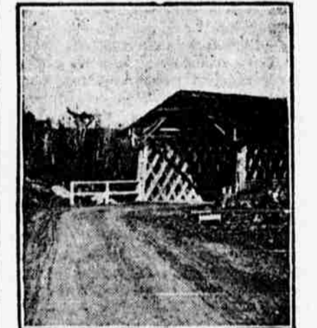
THE SAME ROAD IMPROVED.
