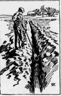
FIG. II-POOR WAT TO LAY TILE.
