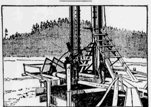
The simple apparatus herewith illustrated is in common use on Canadian rivers during the salmon incubating season. The wheel, placed at the station, arrests the fish on their way down stream and holds them without injury to their delicate bodies. The spawn is then removed from them and put into the incubators. It is a rather crude device, but it seems to answer the purpose as well as the more elaborate process employed on the Columbla River.
