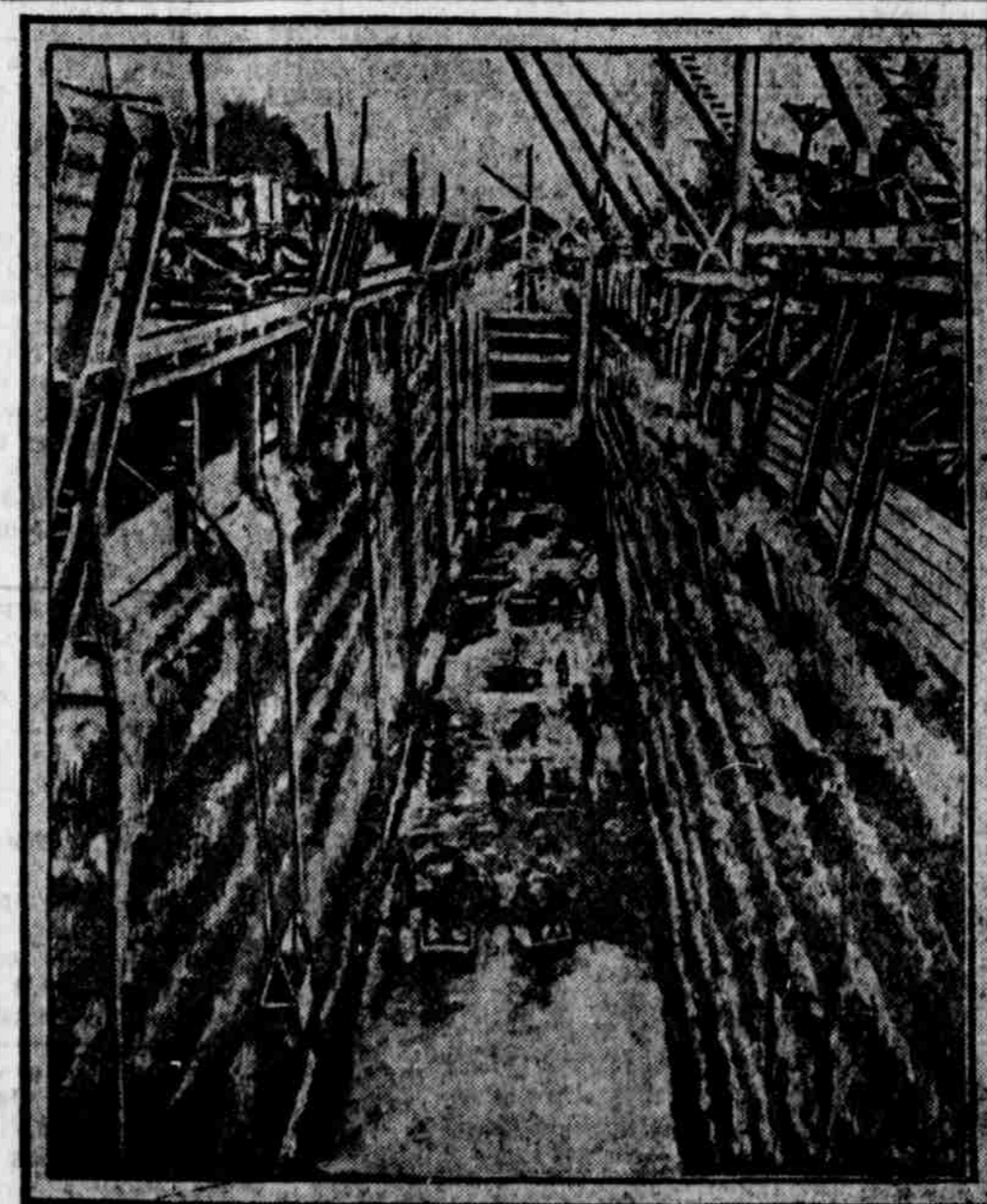
WHEEL PIT OF CANADIAN POWER COMPANY.—From The World To-day.
