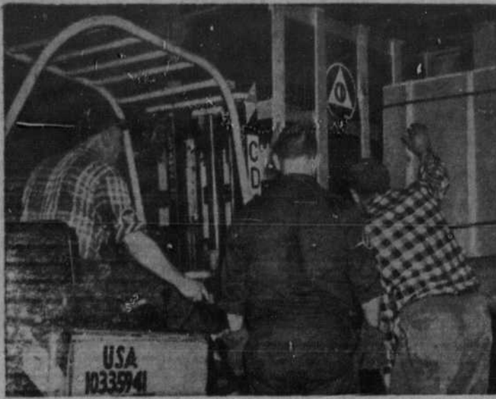
EMERGENCY HOSPITAL 15-kilowatt generator for operating room lights and power equipment is loaded at a Federal Civil Defense Administration warehouse onto two trucks. In attack situations, an entire self-sufficient 13 1/2-ton hospital of 238 items in 450 containers could be moved by a single large truck to a school, church or other suitable building which was reasonably undamaged. (FCDA Photo)
