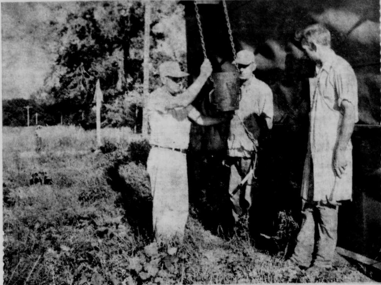
Face Lifting for Old Elevator
