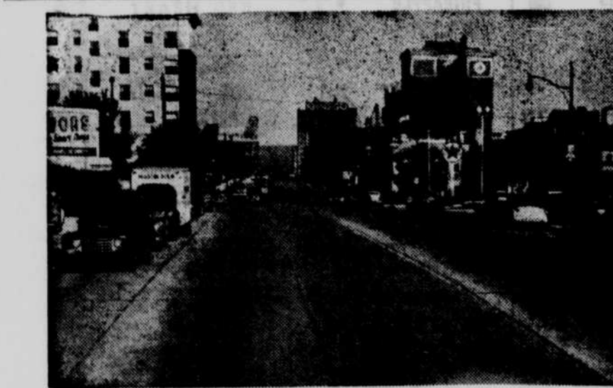
Dodge Street in Omaha. Built in 1948, the pavement is 60 ft. wide.
