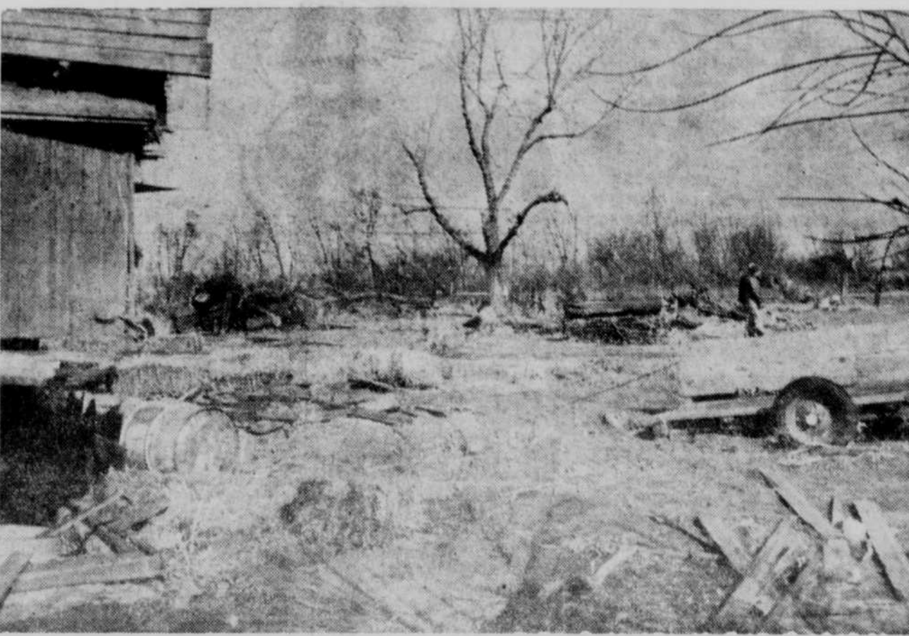
This is a northwesterly view at the Carl Michaels farm in the wake of Monday's tornado. Barn and dwelling were damaged.—The Frontier Photo.
