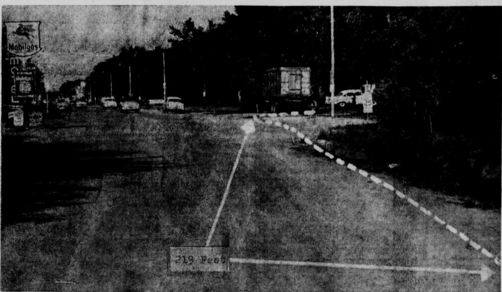
This is the approximate route taken by the McNally truck. The culvert, which is blamed for starting much of the trouble, is barely visible (right center, on dotted line).—The Frontier Photo.
