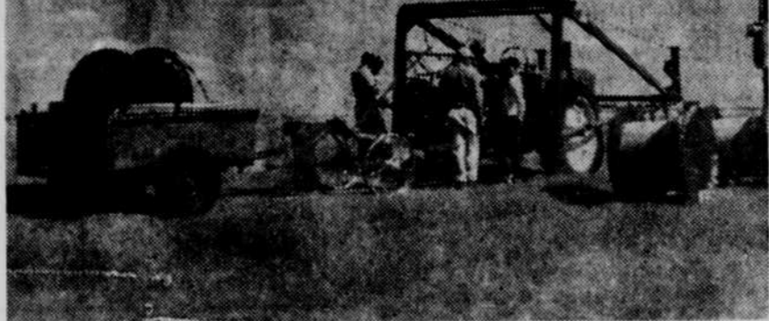
Improved machine constructed by two O'Neill firms lays electric cable for wind testers.—U.S. Air Force Photo.
