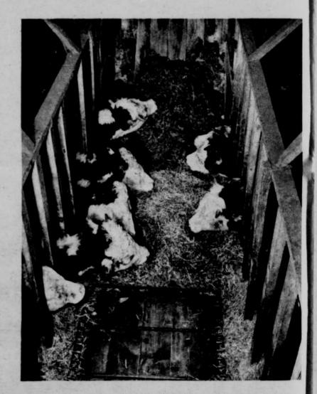
Silage, hay or grain can be fed mechanically in the barn by this apron conveyor bunk. The apron is made from manure spreader parts and can be reversed to carry silage from the silo chute at one end of the barn or hay from the other end. Vertical slats above the bunk prevent fighting for space at the bunk.
