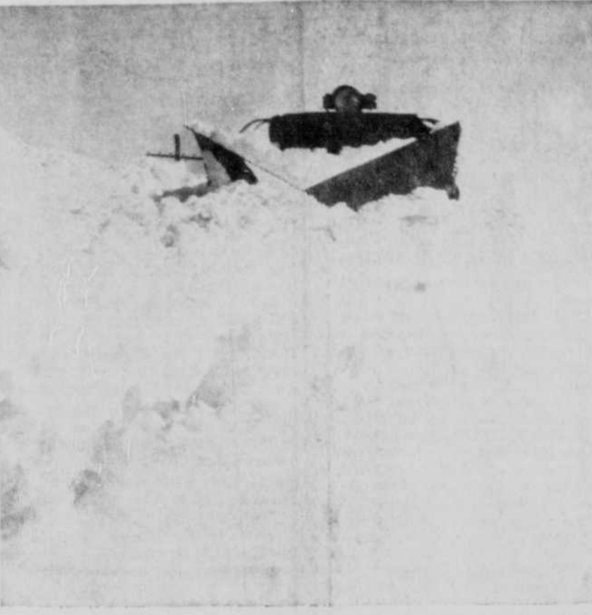
This frontal view of the snowplow, which headed a stranded two-engine Burlington freight train, testifies to the depth of the snow near McLean. The O'Neill-bound freight was liberated Wednesday afternoon after two days in a snowbank. The snow measured from 15- to 20-ft. in depth. Snow in foreground had been removed by bulldozers. Photo was taken a short time before the breakthrough which resulted after two additional engines came from behind to the rescue.—The Frontier photo and engraving
