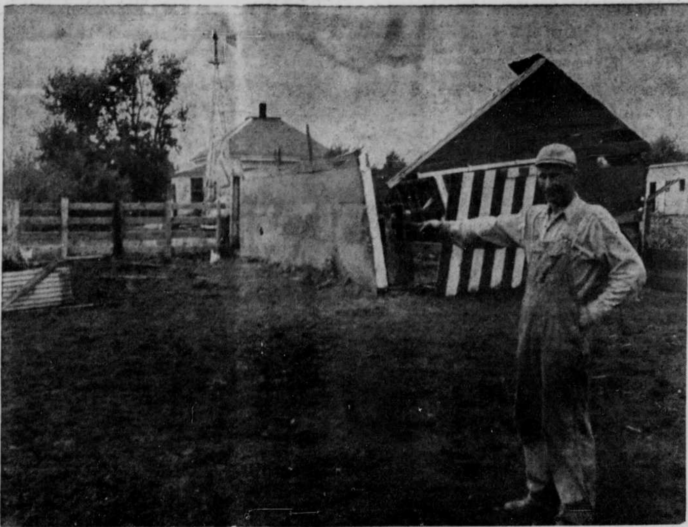
WIND WRECKS HOG SHED... Leo Turay miles northeast of O'Neill. Also damaged were points to a demolished hog shed that yielded ungrain bin, windmill, hay rack and virtually all der Sunday night's tornadic wind. Steel roof roofs on the place.—The Frontier Photo & Engraving.
