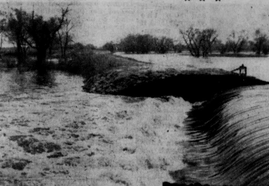
WATER OVER THE DAM . . . The Atkinson mill dam weathered the high water in the upper Elkhorn river last week even though there was considerable apprehension when water neared an all-time high mark. The earthen dam was banked with baled hay to secure it. This graphic photo showing water racing over the spillway was taken on Tuesday, May 15.—The Frontier Photo to Elwood Brady.
