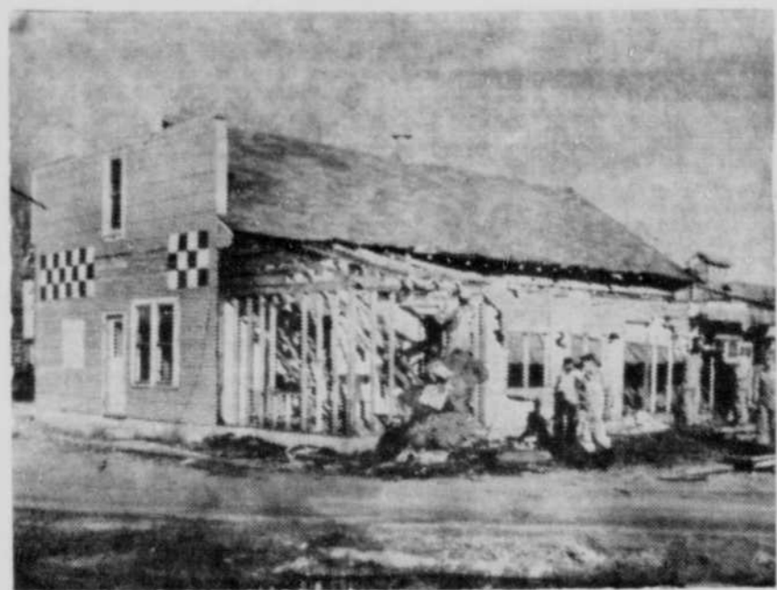
Portion of Building Comes Down
