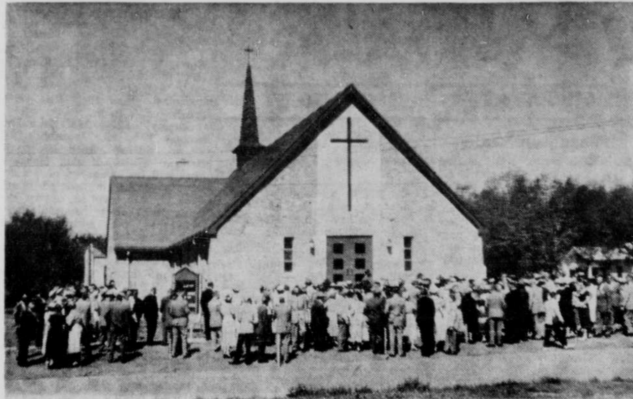
This photo of the new 76-thousand-dollar Christ Lutheran church was taken Sunday morning moments before the doors were formally opened for the first time. The main part of the church and the basement overflowed with parishioners, former members of the parish, visitors and other well-wishers.—The Frontier Photo.
