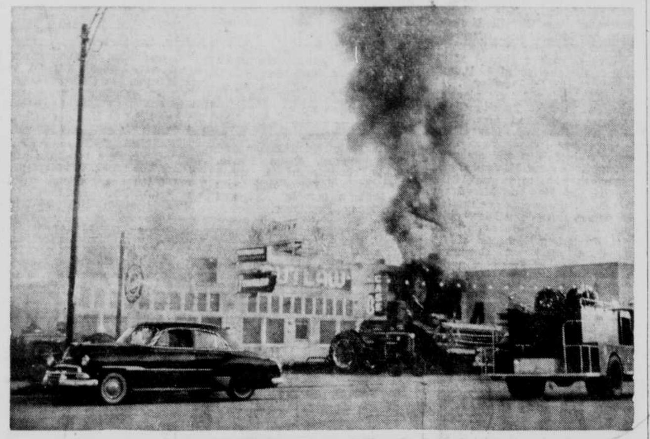
Smoke and flames emerge from the front of the Outlaw Implement company building during the early phases of the Saturday night fire which caused an estimated 30- to 40-thousand-dollar damage.—The Frontier Photo.
