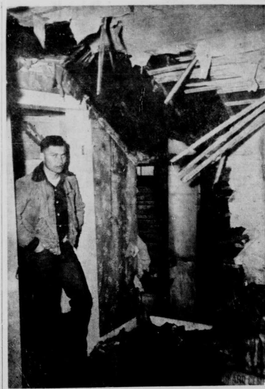
Farm Home Damaged by Fire
