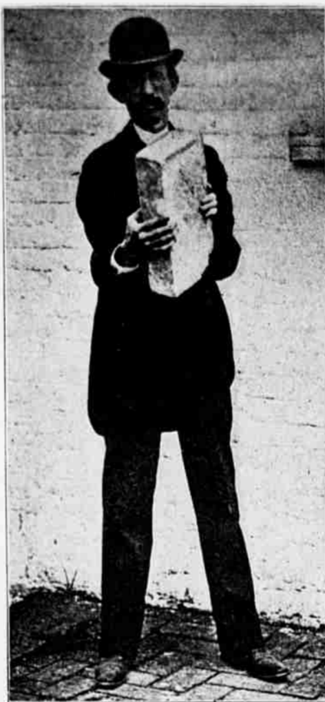
FRANK G. CARPENTER HOLDING UP A BRICK AT THE GREAT WALL OF CHINA TO SHOW ITS SIZE.
