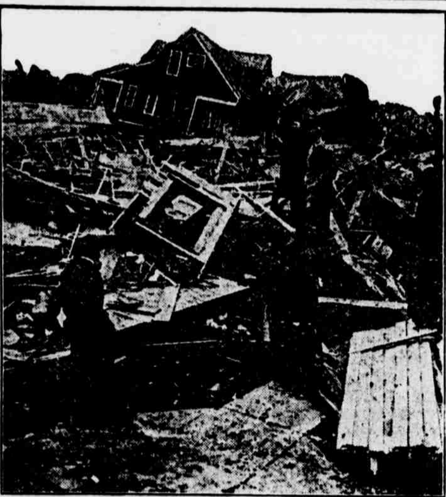
The devastation caused by the Omaha tornado is graphically illustrated by this photograph, taken at Lincoln boulevard and Thirty-fourth street, directly in the path of the storm.
