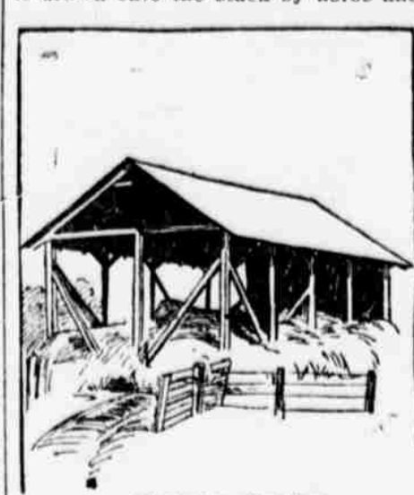
Shed for Feeding.
