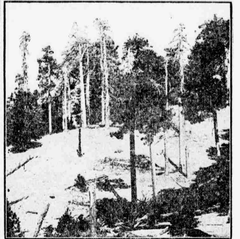
Logged, Burned and Grazed Slope.
