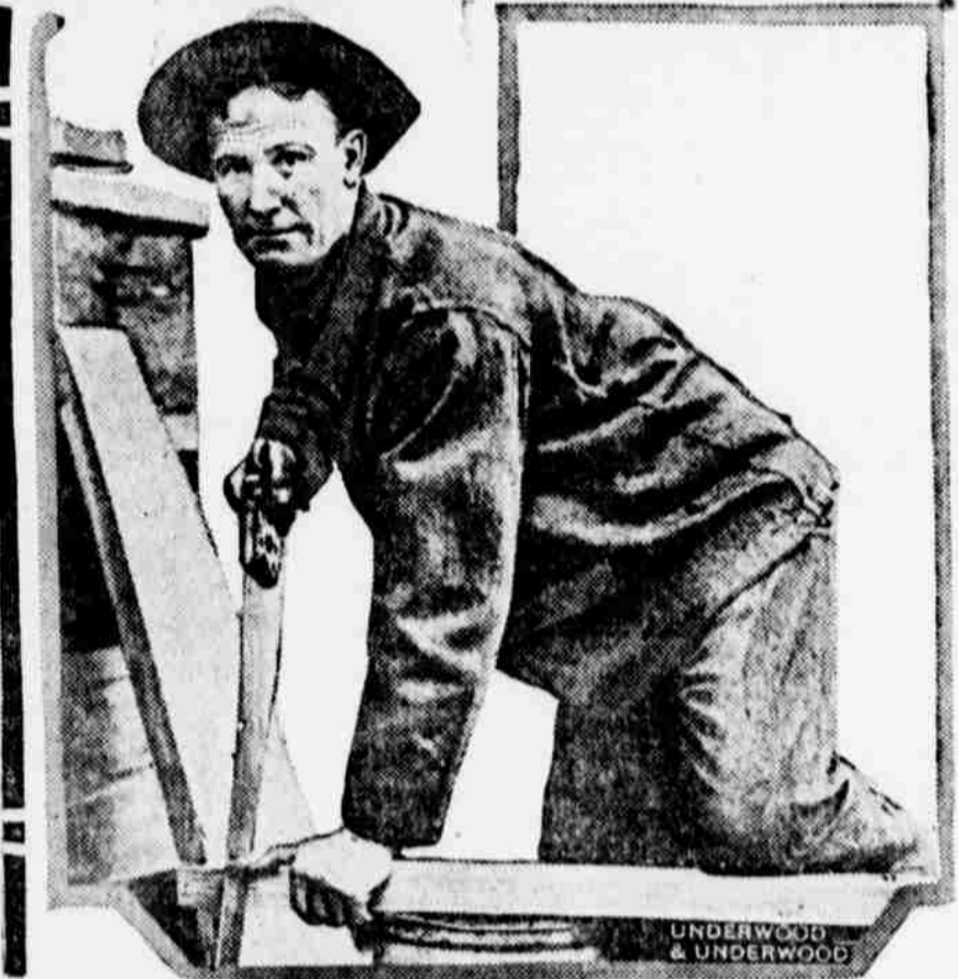
General Pershing chose him as the greatest single hero of the World war, but that honor does not prevent Sergeant Samuel Woodfill from going to work on a dam for $8.00 a day. He is one of the carpenters at work on the government dam at Silver Grove, Ky. "My husband went to work on the dam because he finds it necessary to raise money to meet the payment on our home that will soon fall due," Mrs. Woodfill said. "He could never do it on his sergeant's pay and the work at the dam opened a way for him."
