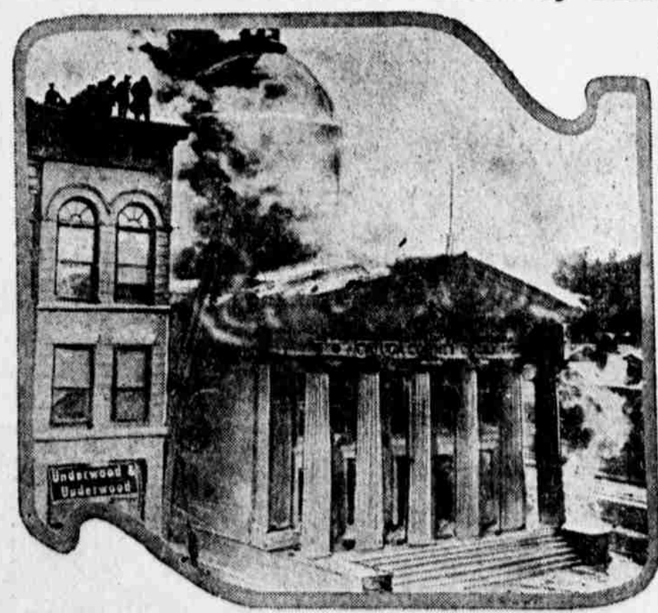
Firemen in Auburn, New York, fighting the flames, which gutted the Cayuga county court house, a venerable building of classic beauty erected in 1836. The cupola, roof and courtroom were totally wrecked.
