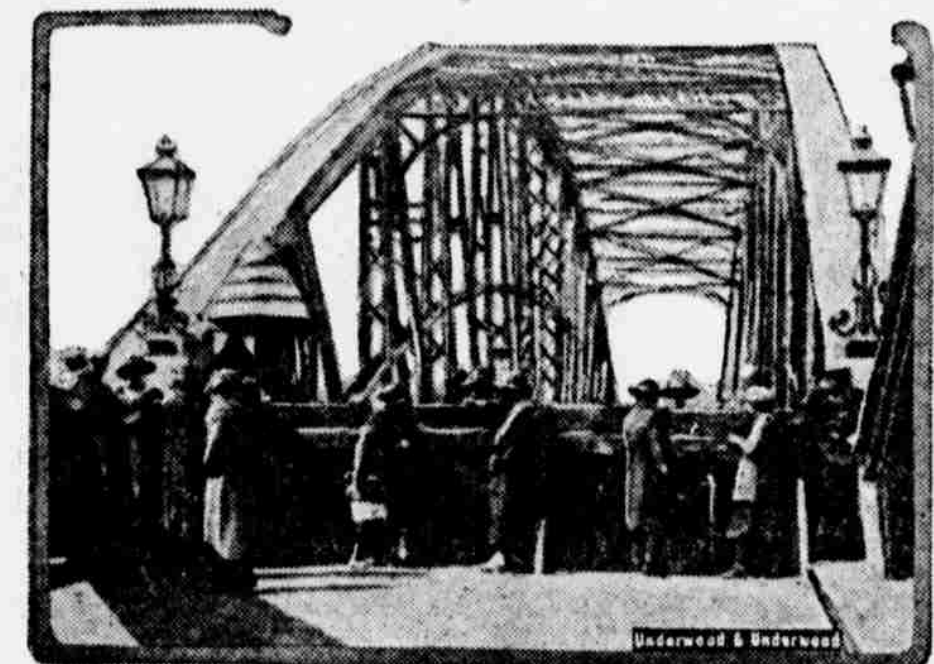
Only at certain hours on Sunday may persons cross this bridge, and then under strict supervision, for it is the bridge between Hungary and Czechoslovakia, over the Donau river, at Extergon, Hungary.
