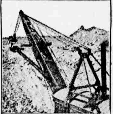
Legion Men Operating Steam Shovel.
