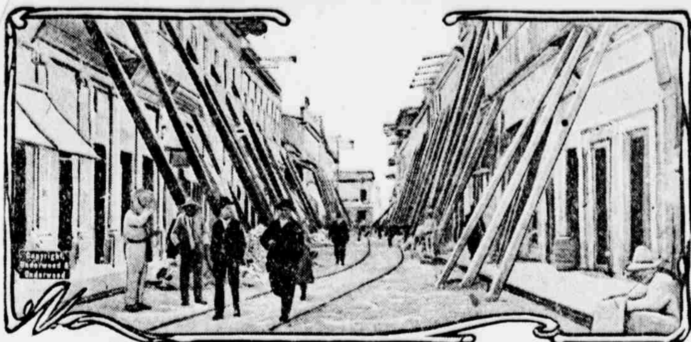
Buildings in Jalapa, capital of the state of Vera Cruz, Mexico, thrown out of plumb by the recent earthquake, are shown propped up to prevent collapse. Vehicular traffic has been suspended on the thoroughfares thus affected for fear the least vibration would bring the weakened buildings down.
