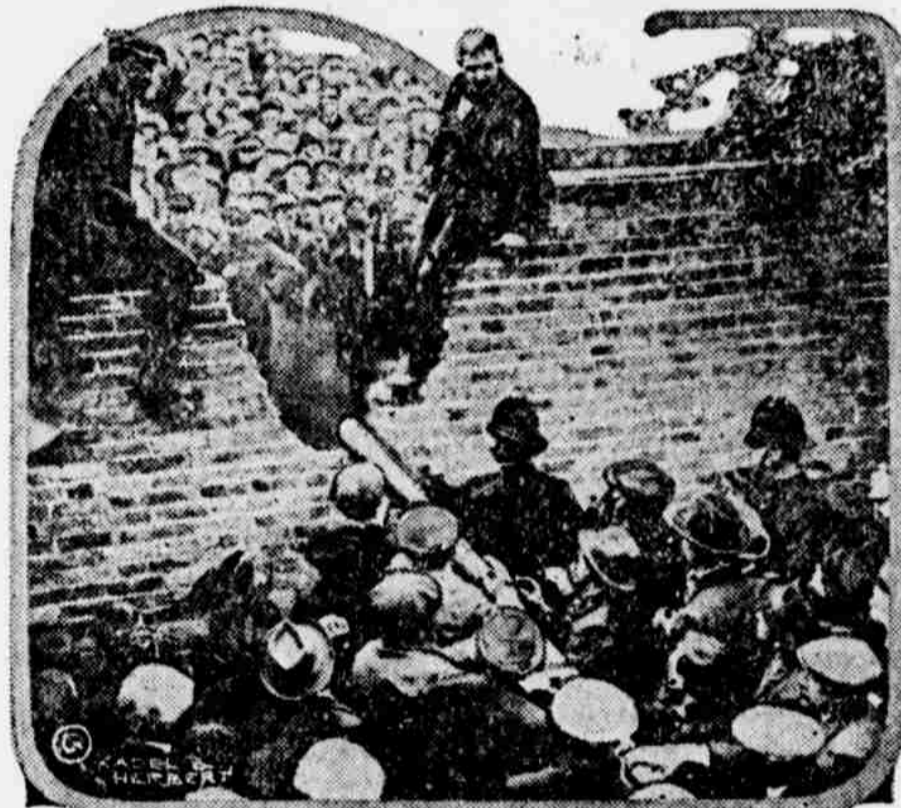
The British citizen always has been most jealous of the maintenance of his ancient rights of way. In order to re-establish their right of way through a bridal path leading to Hanworth park, the residents of Feltham, Middlesex, marched through, demolishing a wall en route. The path had been closed for a government aerodrome.
