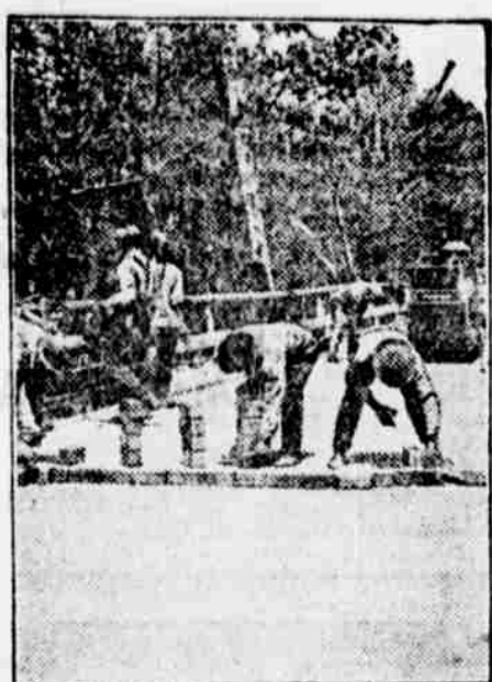
Laying Vitrified Blocks.
