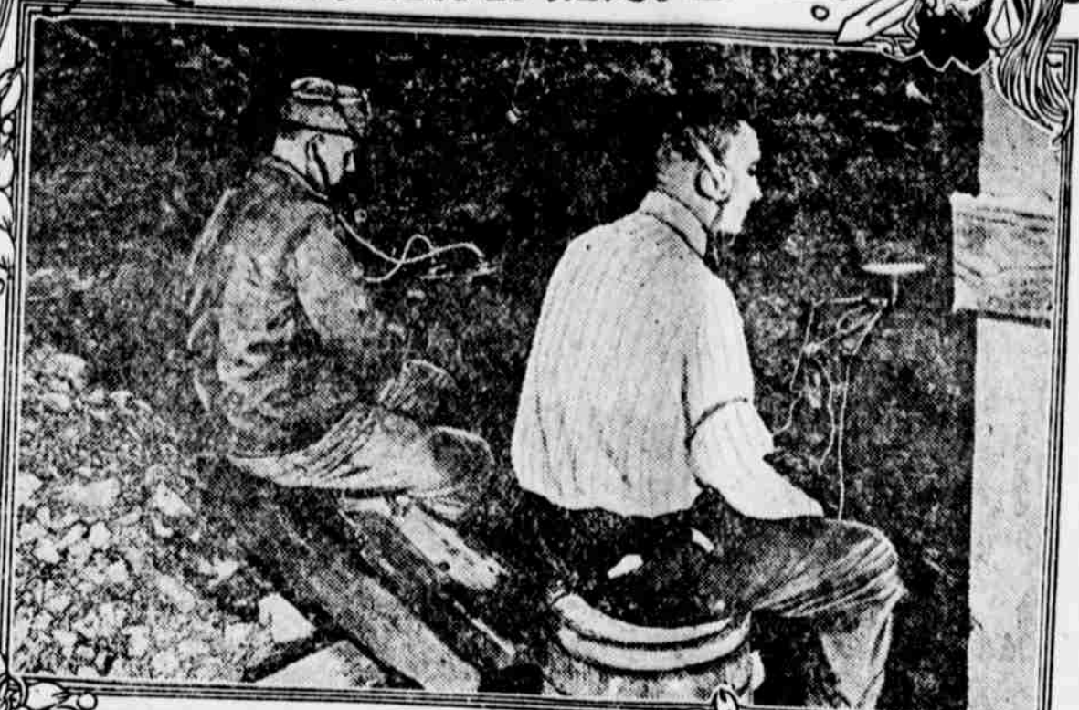
MINING RESCUE GEOPHONE SET LISTENING TO EXPLOSION OF ONE OUNCE OF DYNAMITE 1/2 MILE AWAY
