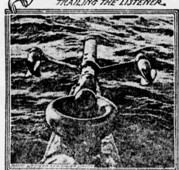
LISTENING DEVICE ON PROW OF SUBMARINE
