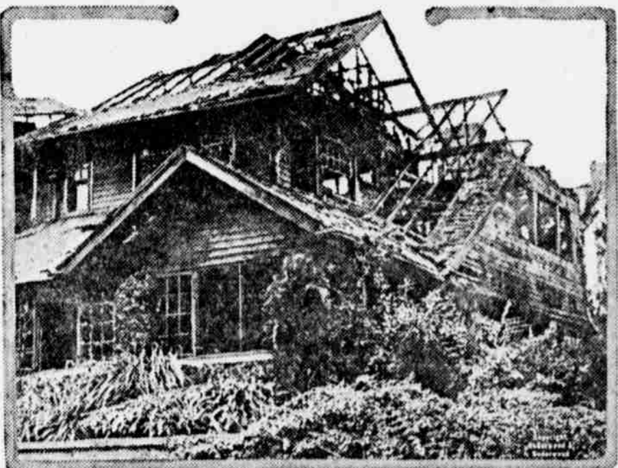
Ruins of home of Oscar Lawler, Los Angeles, Cal., which was blown up by a dynamite bomb and fired with two tanks of gasoline. Mr. Lawler was assistant United States attorney general for the interior department. Charles H. McGuire was accused of setting the bomb in revenge for the breaking of a will by Attorney Lawler. He committed suicide.
