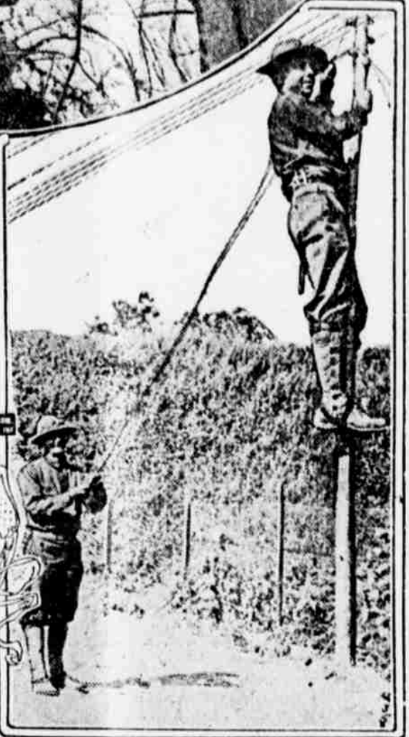
AMERICAN LINEMEN STRINGING WIRES BEHIND LINES
