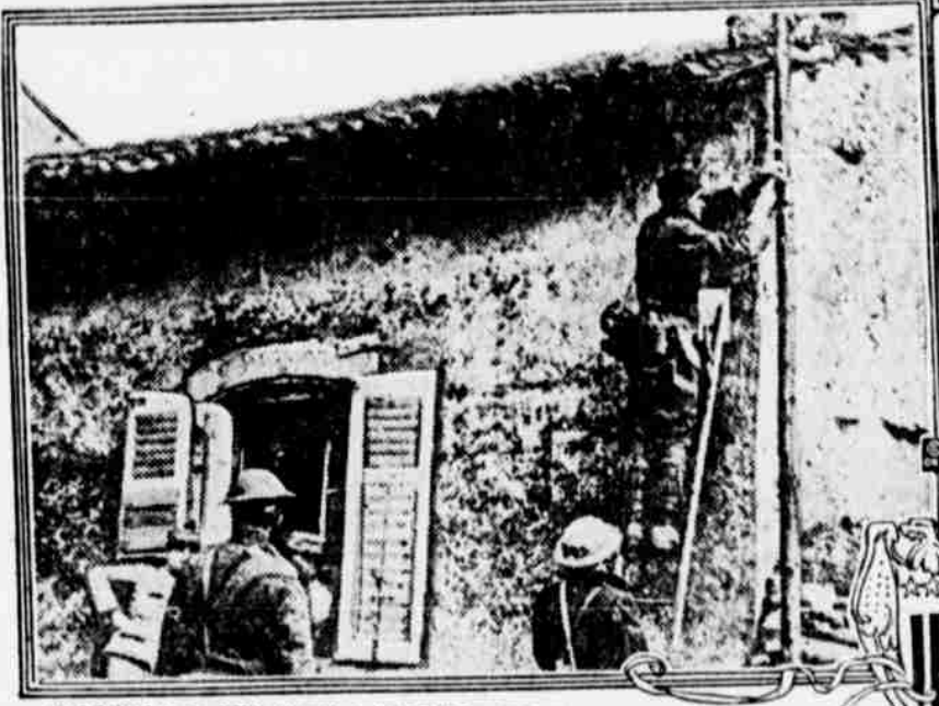
REPAIRING BROKEN LINE "SOMEWHERE IN FRANCE"
